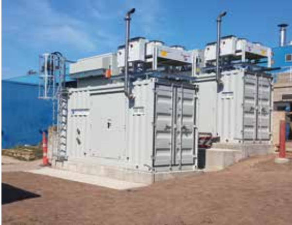
Twin KB 100 Biogas CHP Modules Pictured above
